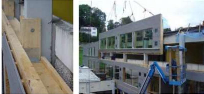
Figure 8 School in Schwanenstadt: installation of facade elements
